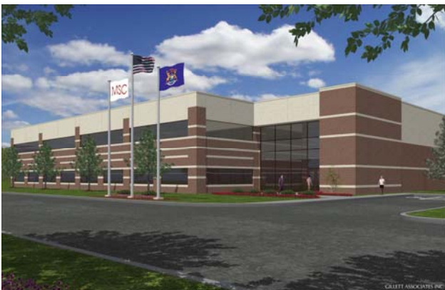
Application Research Center (ARC)
